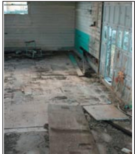
Figure 2.34 High bay of Building #9, looking west
