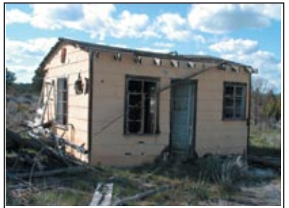
Figure 2.46 Building #23, Trailer Court Utility House, Southeast Corner
