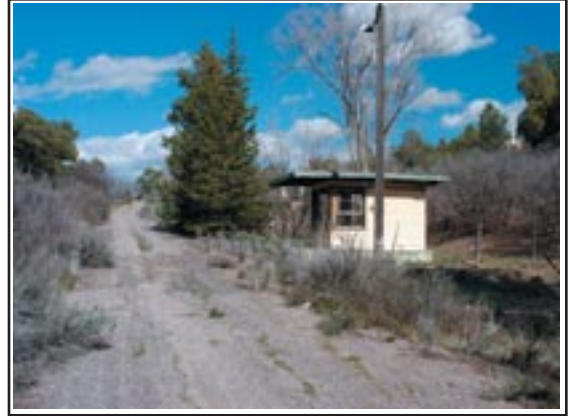
Figure 2.32 West facade of Building #8, Guard House
