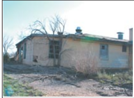
Figure 2.29 East end of south facade of Building #7
