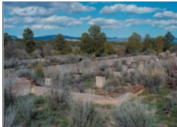
Figure 2.27 Foundation of Building #6, Officers Quarters
