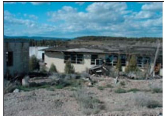
Figure 2.33 South facade of Building #9, Recreation Facility/Squadron Headquarters
