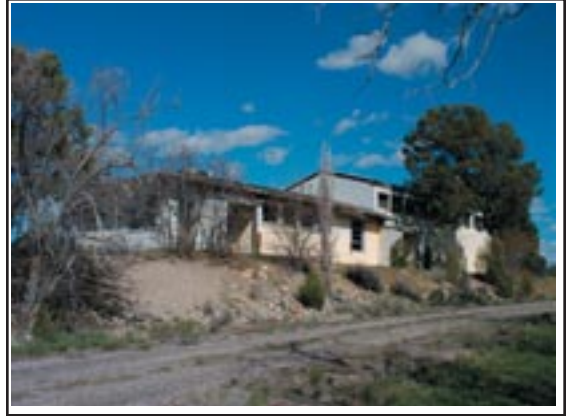
Figure 2.44 Building 22, Recreation Facility, Southwest Corner
