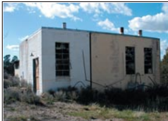
Figure 2.19 East Facade, Building #4, Heating Plant
