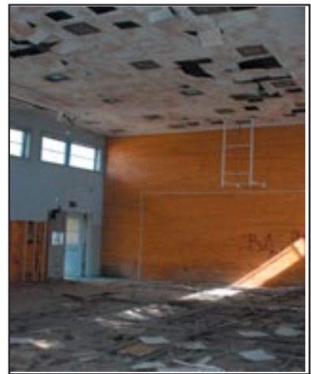
Figure 2.45 Building 22, Recreation Facility, Multi-Purpose Room
