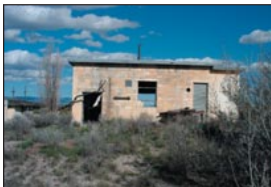
Figure 2.16 West Facade, Building #2, Electric Primary Power
