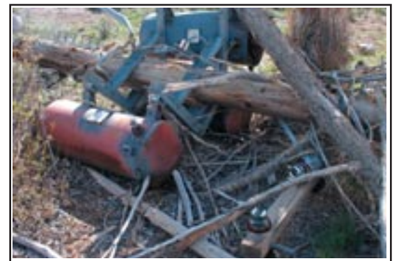
Figure 2.10 Remains of a pole mounted electric transformer
