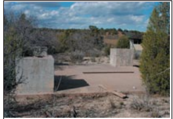
Figure 2.9 Foundation of Radar Tower
