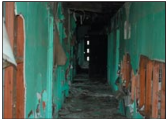
Figure 2.25 Interior Corridor, Building #5-B, Airmen's Dormitory
