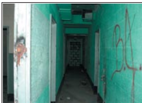
Figure 2.15 Corridor of Building #1, Operations
