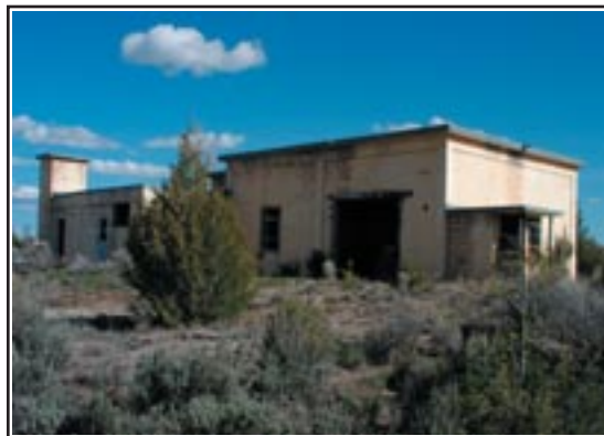
Figure 2.14 Northwest corner of Building #1, Operations
