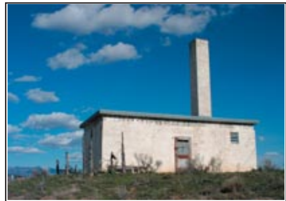
Figure 2.39 Building #12, Communication Receiver
