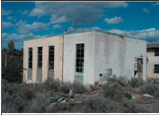
Figure 2.20 West Facade, Building #4, Heating Plant
