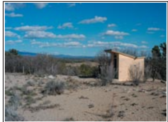
Figure 2.47 Builidng #25, Paint Storage Building, West Facade
