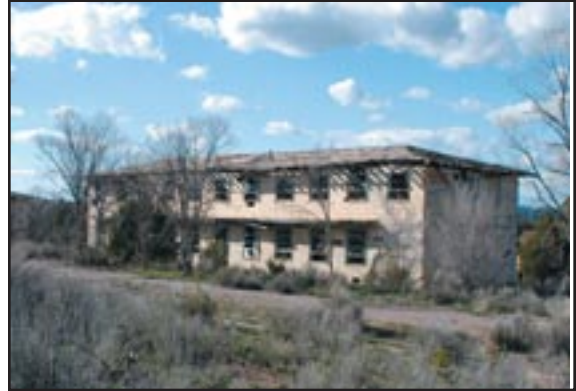
Figure 2.23 Southeast Corner of Building #5-A, Airmen's Dormitory
