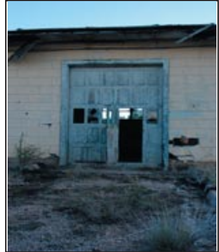
Figure 2.35 North facade, west end of Building #9, overhead door
