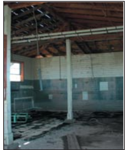
Figure 2.42 Building #14, Supply and Issue Shop Work Bay
