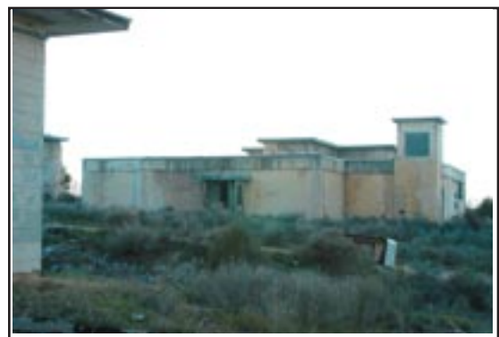
Figure 2.13 Building #1, Operations, East Facade
